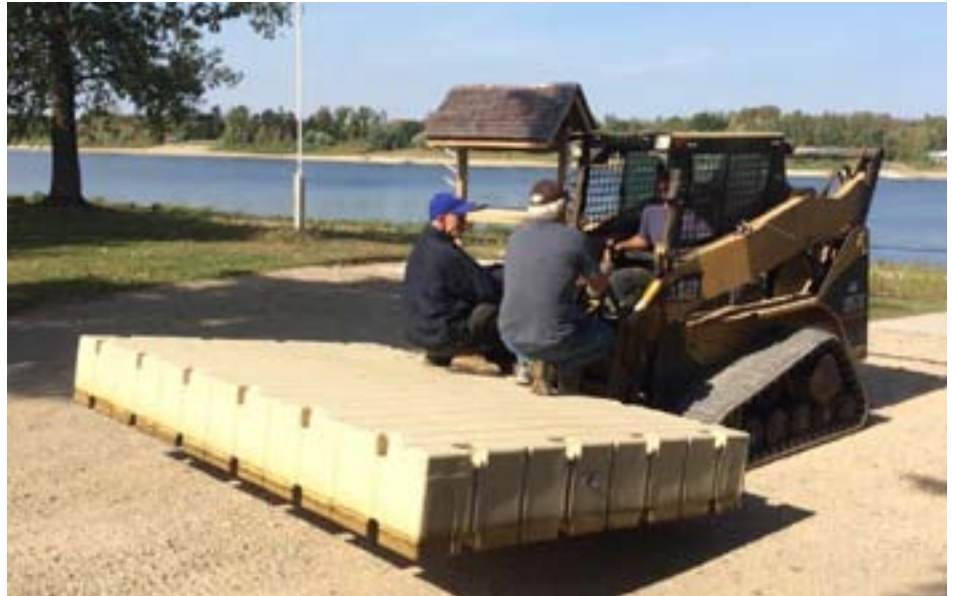
Moving a Section of the New Dock, Club Closing Day 2015
